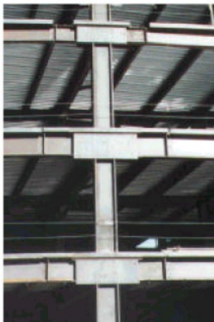
Figure 5: Completed erection of SidePlate™ Connection System.
