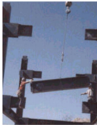
Figure 2: Column Tree/Link Beam erection.
