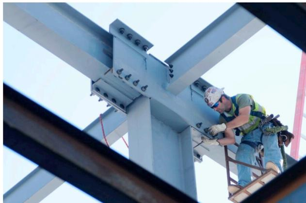
The SidePlate Bolted connection qualifies as a Special Moment Frame (SMF), per the ANSI / AISC 341-10 specification: "Seismic Provisions for Structural Steel Buildings."
