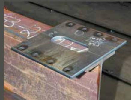
Closeup shows cover plate of moment-connection beam before bolts have been inserted through pre-drilled holes.
